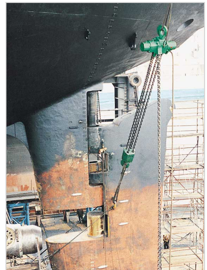
Mounting a rudder blade with two JDN Air Hoists PROFI 100 TI.
